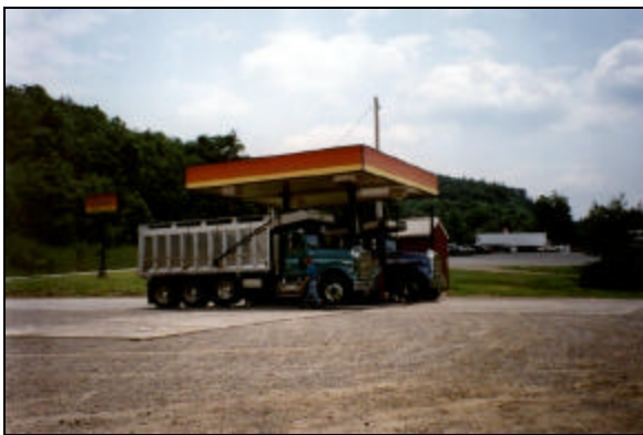
Card-Access Fleet Fueling Station
